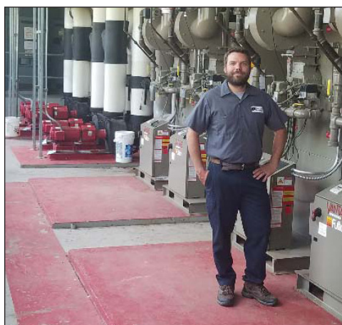
Tim Geets, LEED HVAC technician at River City Mechanical, in front of the Fulton Vantage 4,000,000 BTU boilers at East Kentwood High School.
