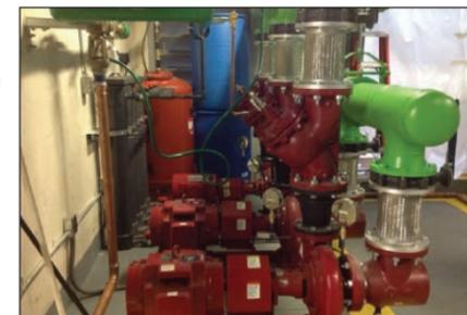
At Annapolis — now known as Oakwood-Wayne — upgrades involved removing one chiller, re-piping existing lines to new and remaining chillers and adding variable frequency drives (VFDs) to the system.
